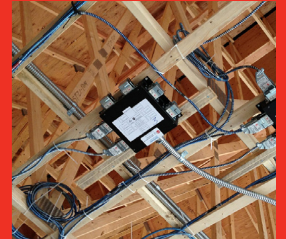
Fastlane Plug N Play systems provides power to all areas of store.
